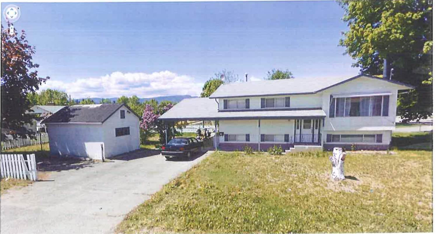
820 Quigley Road, Facing North-West to the property
